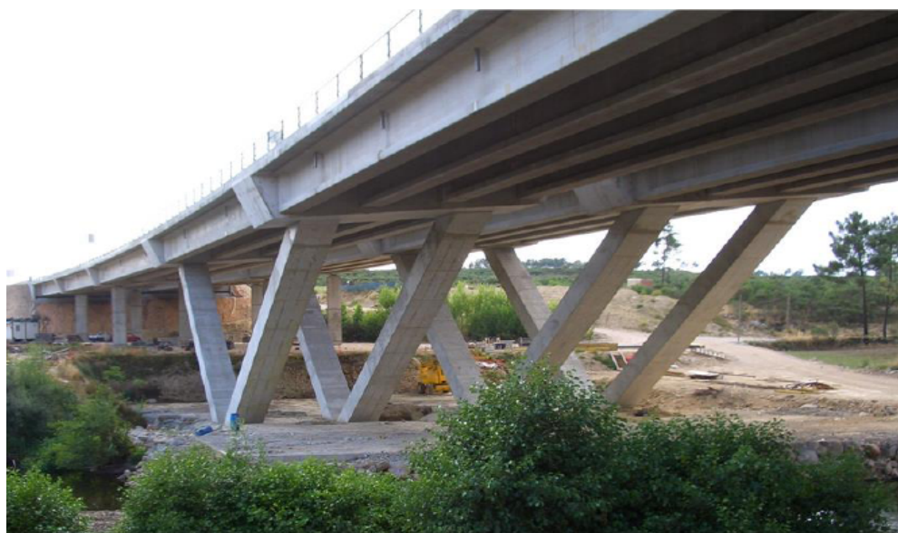
Figure 1.5 Continuous bridge with precast I-girder, courtesy D.H. Ordonez
